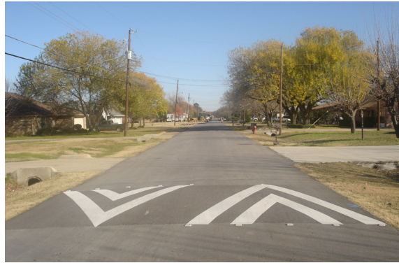
Speed controls like speed humps (left), speed tables, and raised crosswalks (right, pictured in front of Princeton Station) can help control vehicle speeds on shared roadways.
