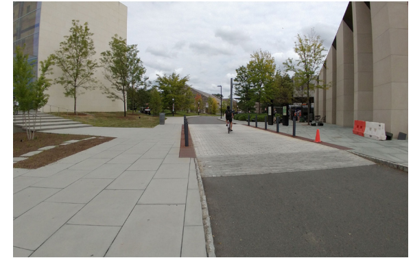
Speed controls like speed humps (left), speed tables, and raised crosswalks (right, pictured in front of Princeton Station) can help control vehicle speeds on shared roadways.
